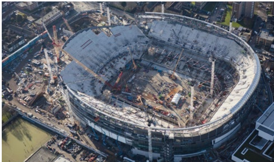
Tottenham Hotspur’s new stadium under construction.
