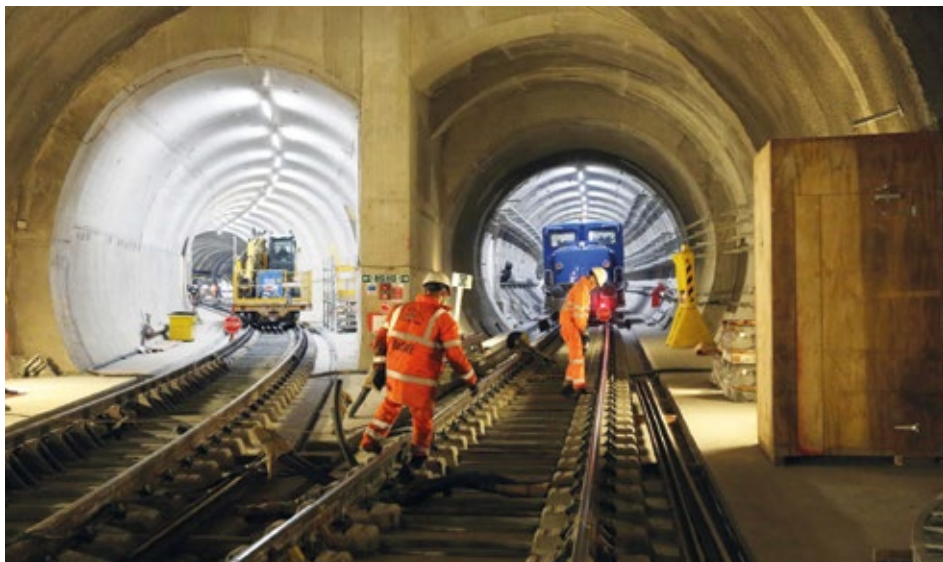
Workers continue track tests in Crossrail tunnels.
